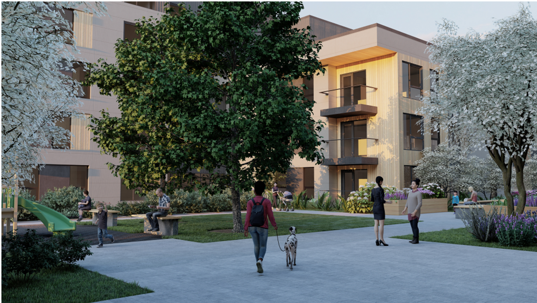
3 View South-West - Thru Courtyard
