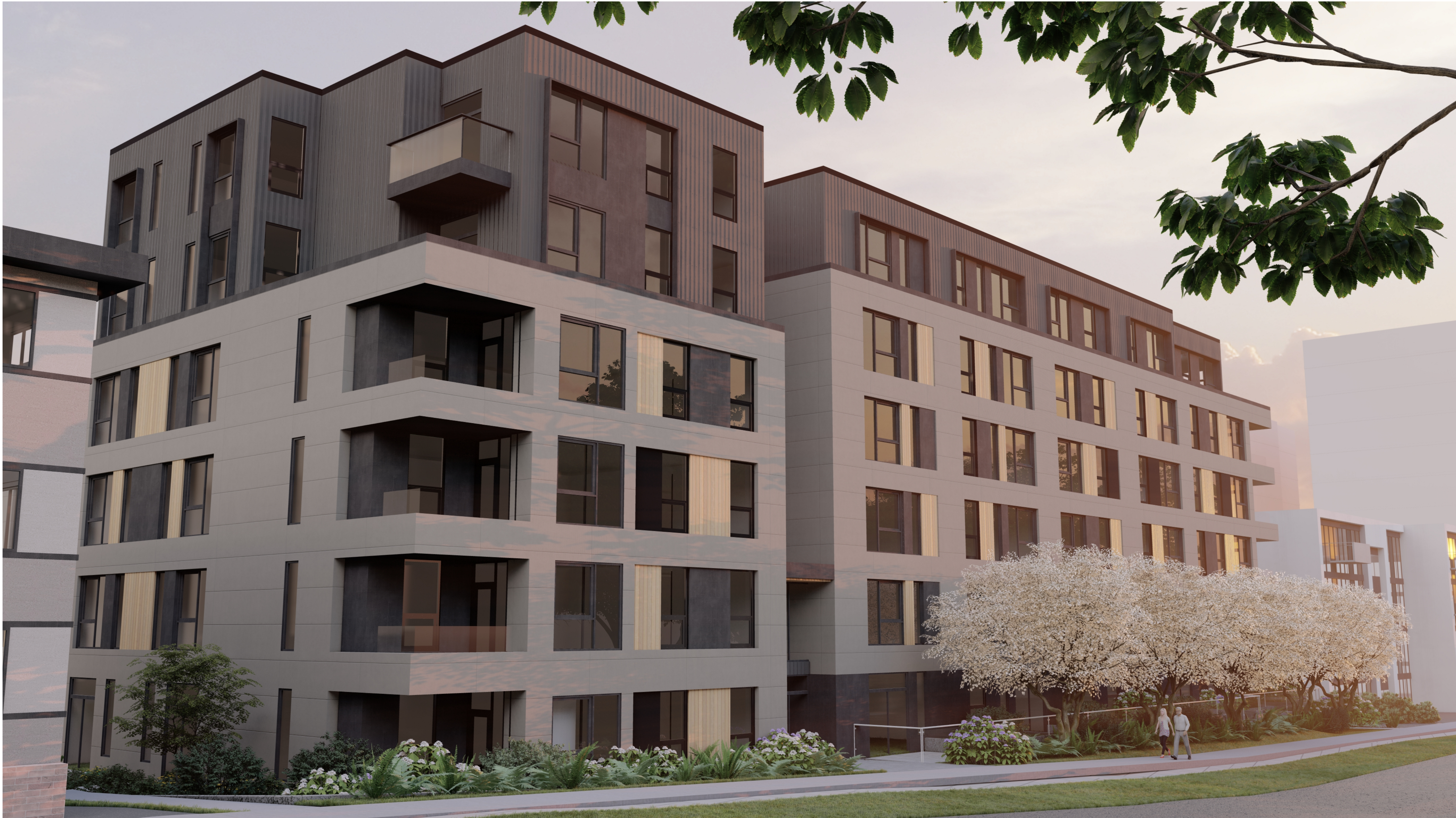
4 North-East Corner View - Pandora St.
