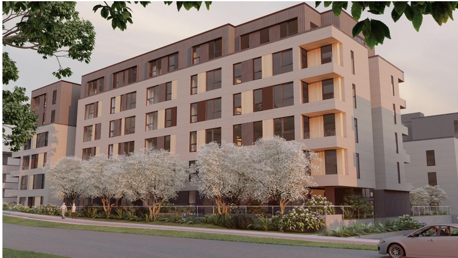
1 North-West Corner View - Pandora Ave.
