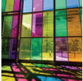
Window Wall System w/ Low E Insulated Glass & LED Coloured Backlit Feature Wall
