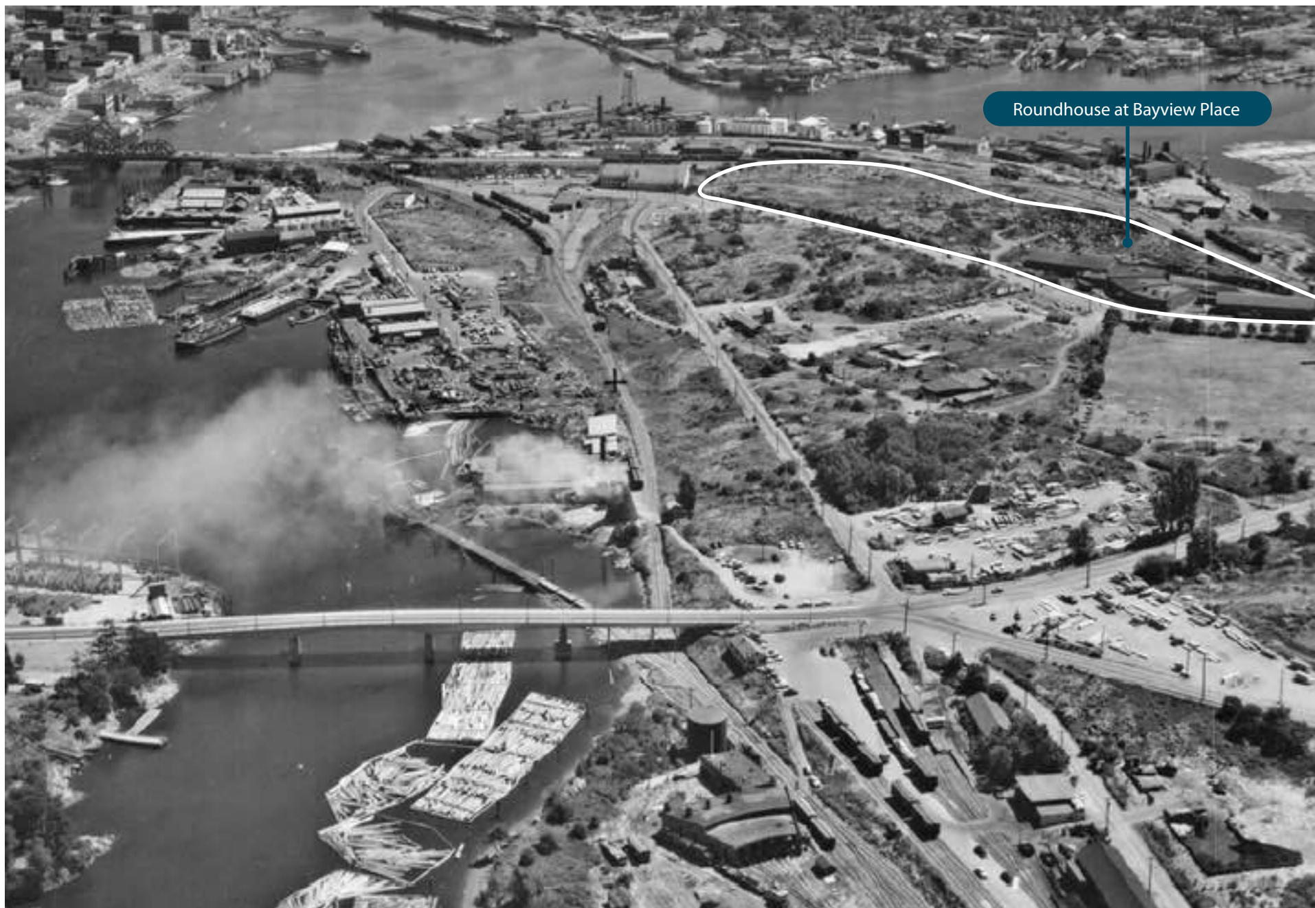
Aerial Photo of Roundhouse at Bayview Place Site
