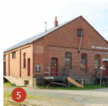
Stores building, view from east (Focus Equities)
