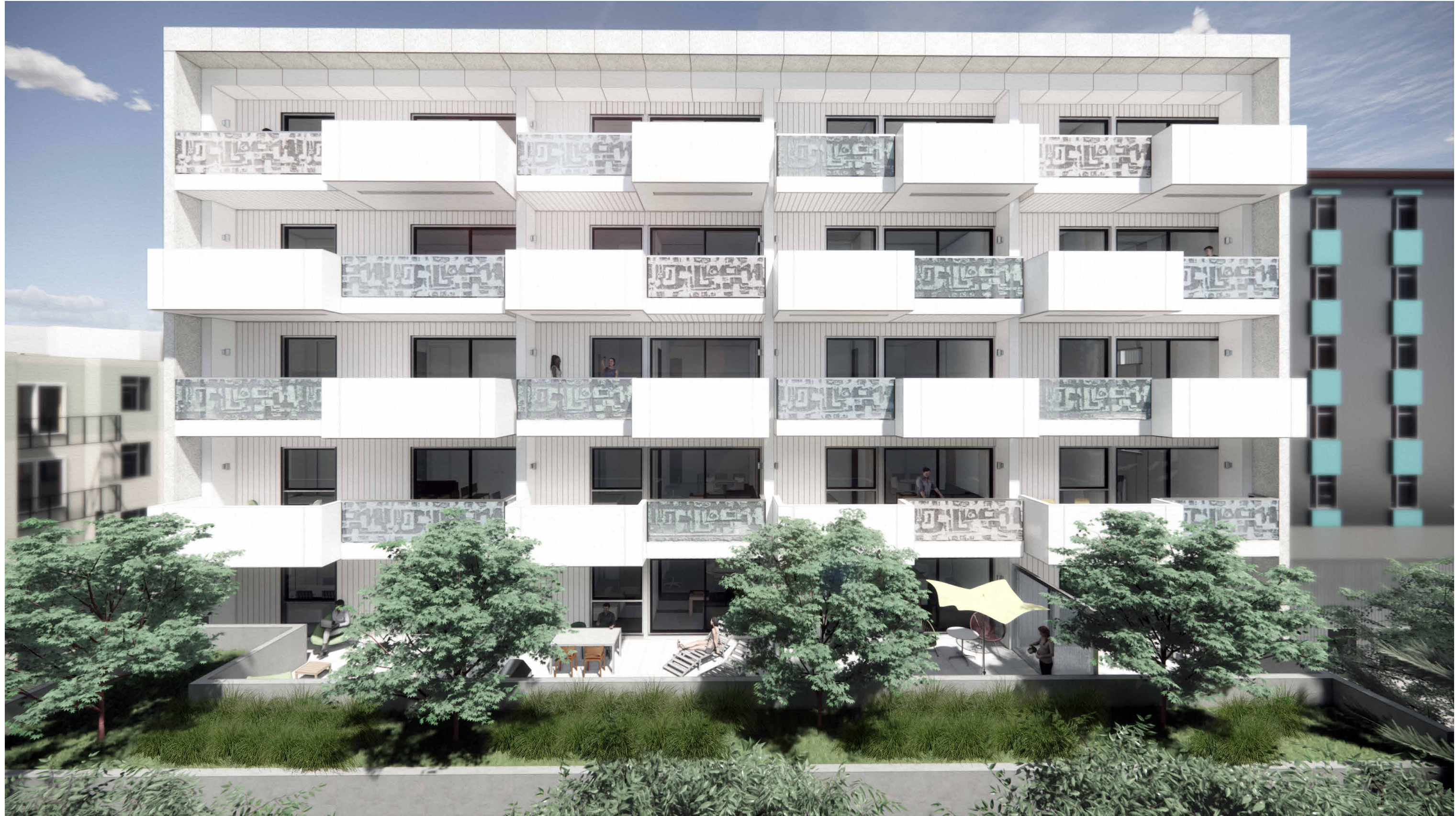
VIEW OF SOUTH FACADE
