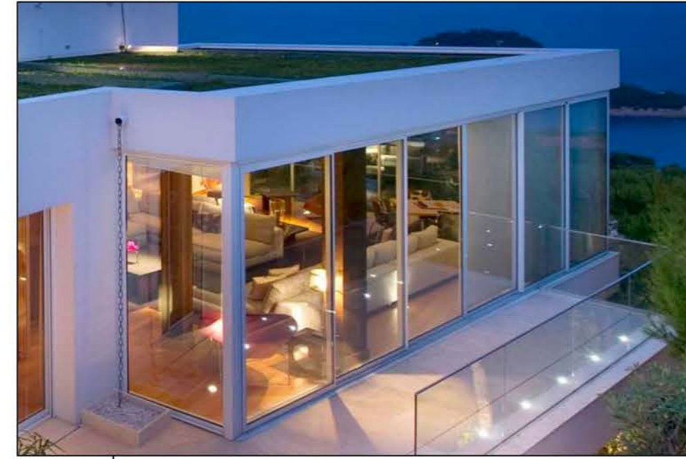
High-Performance aluminium and glass window-wall system
