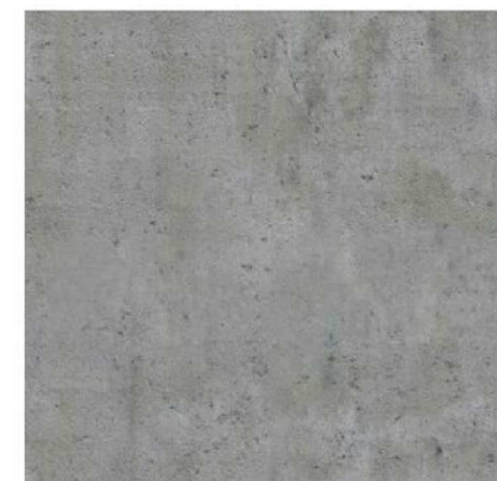
4.1 ▲ EXPOSED CONCRETE FIRE-HALL L1 / SITE
