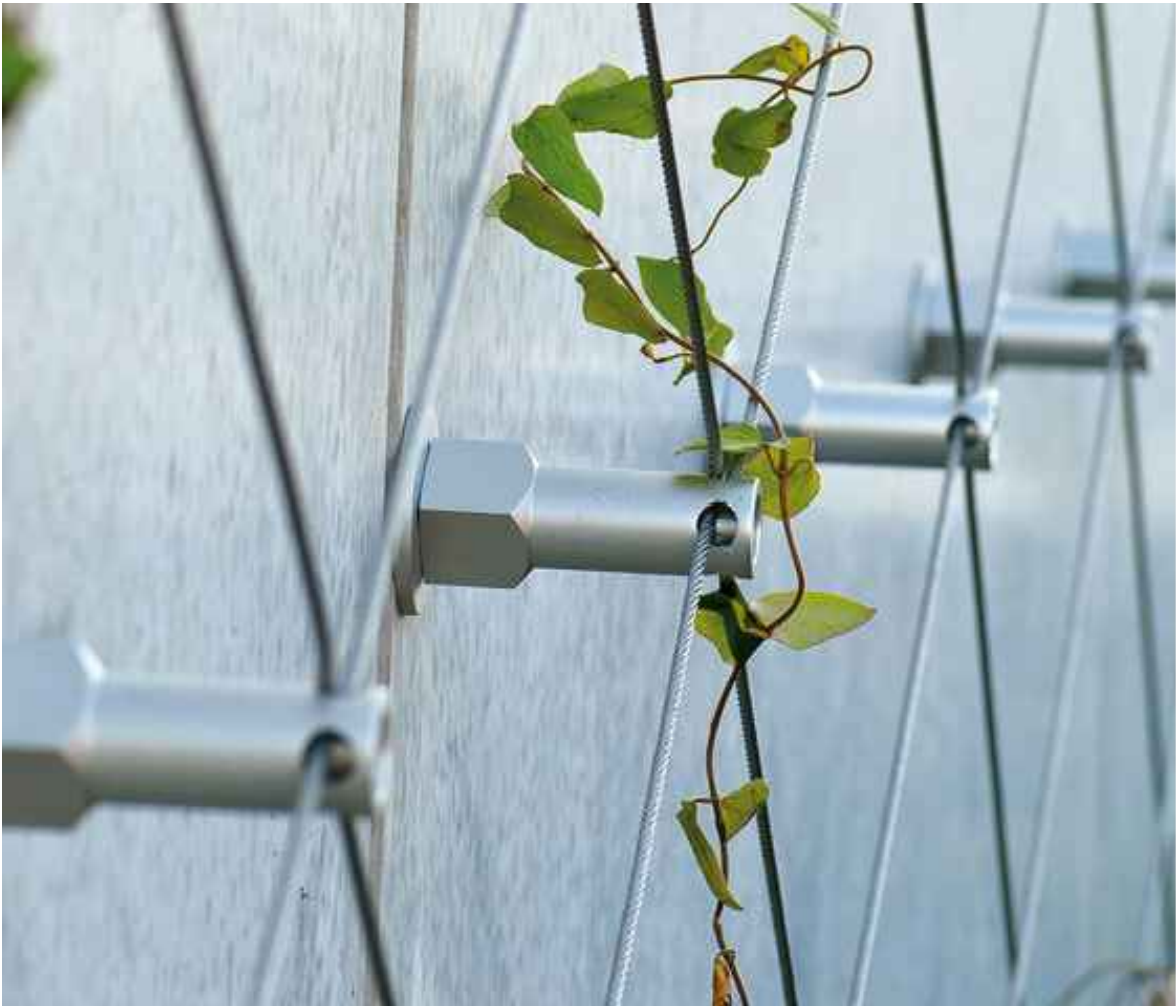
CABLE TRELLIS DETAIL
