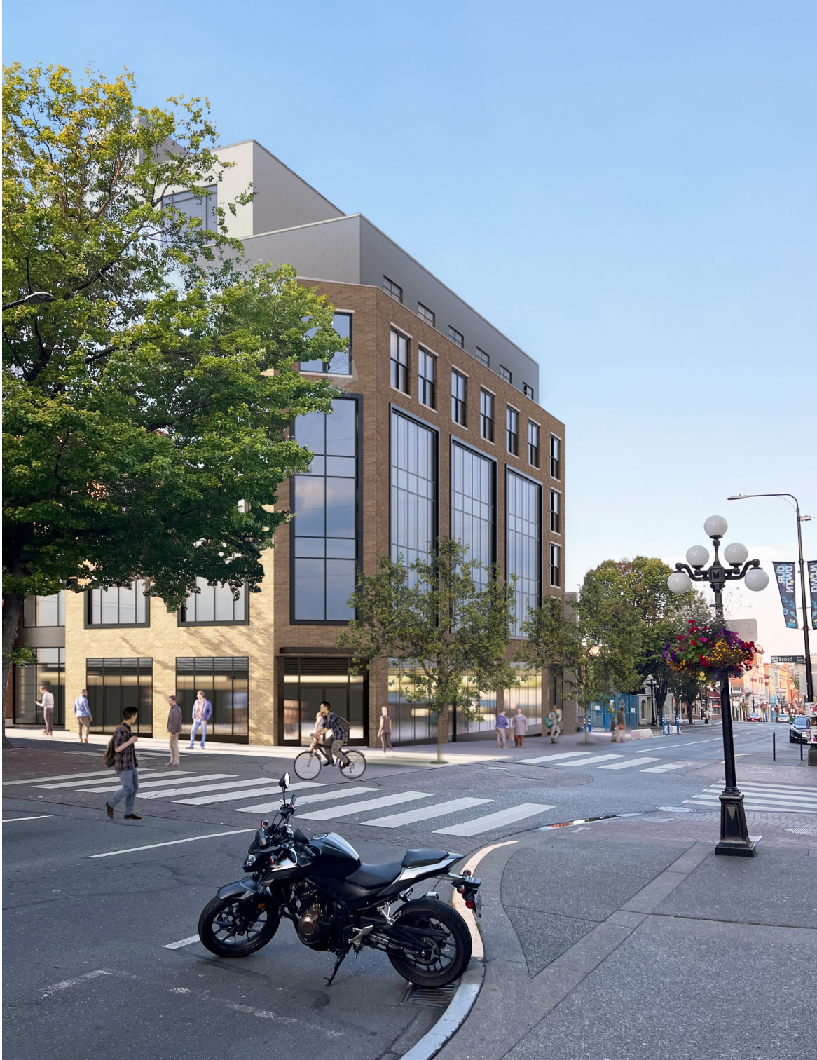
Looking west along Johnson St. towards site.
