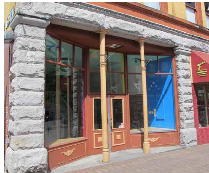
View of Existing Ducks Building storefront on Broad Street.
