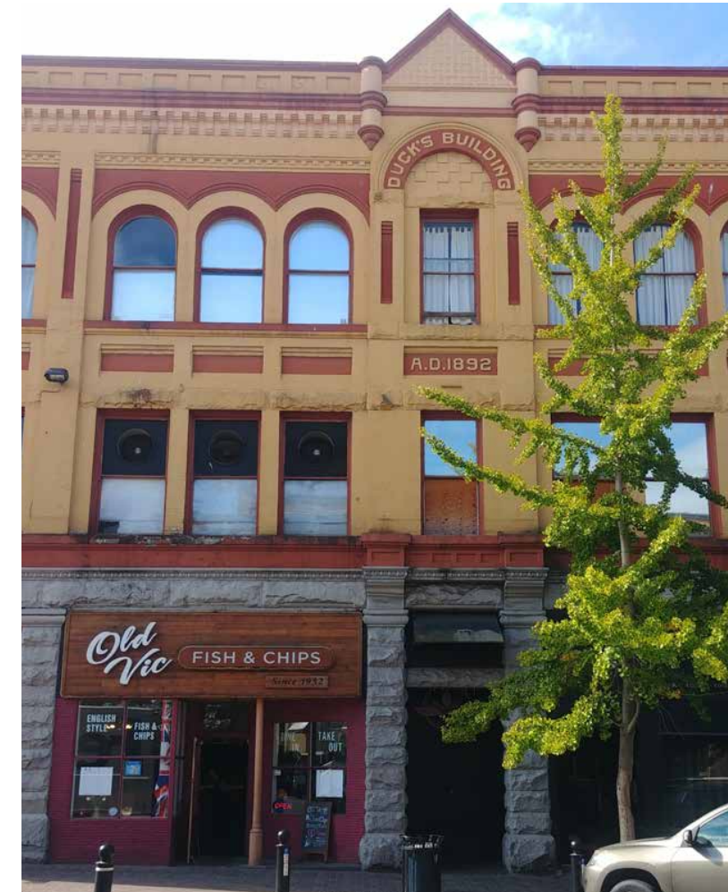
View of Existing Ducks Building storefront on Broad Street.
