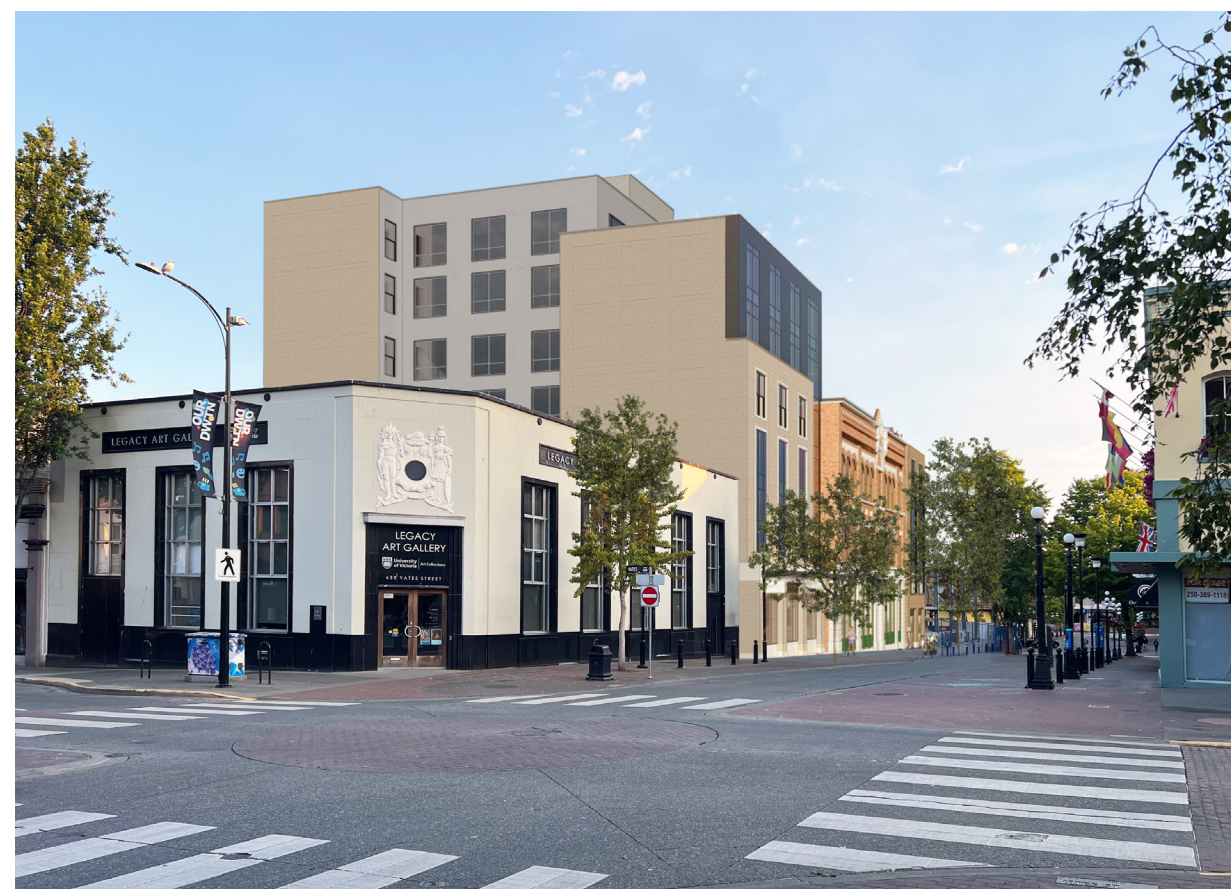
Looking north along Broad St. towards site.
