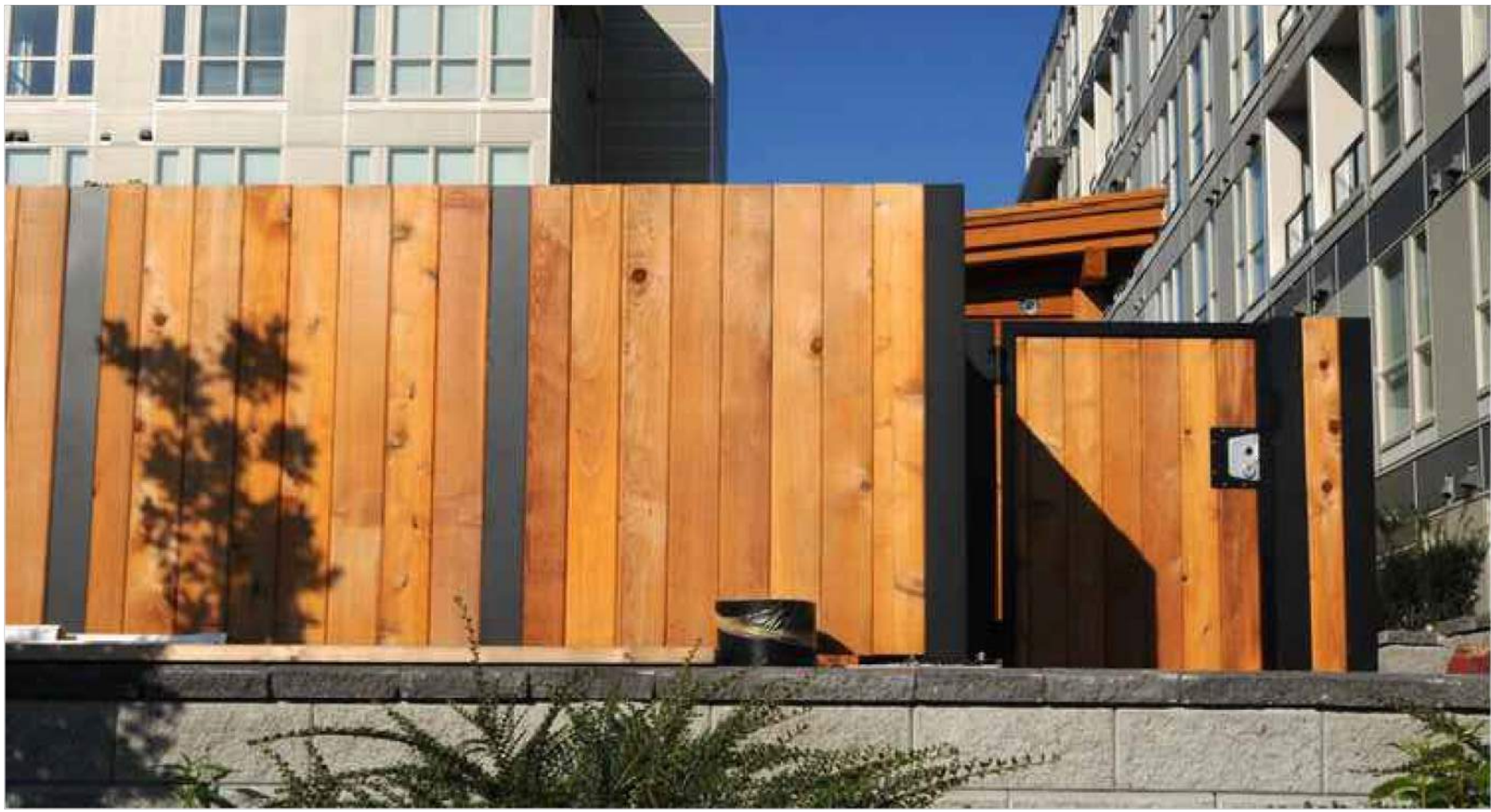
IMAGE 01 - 6' (1.8M HIGH) NON CLIMBABLE FENCE AND GATE
