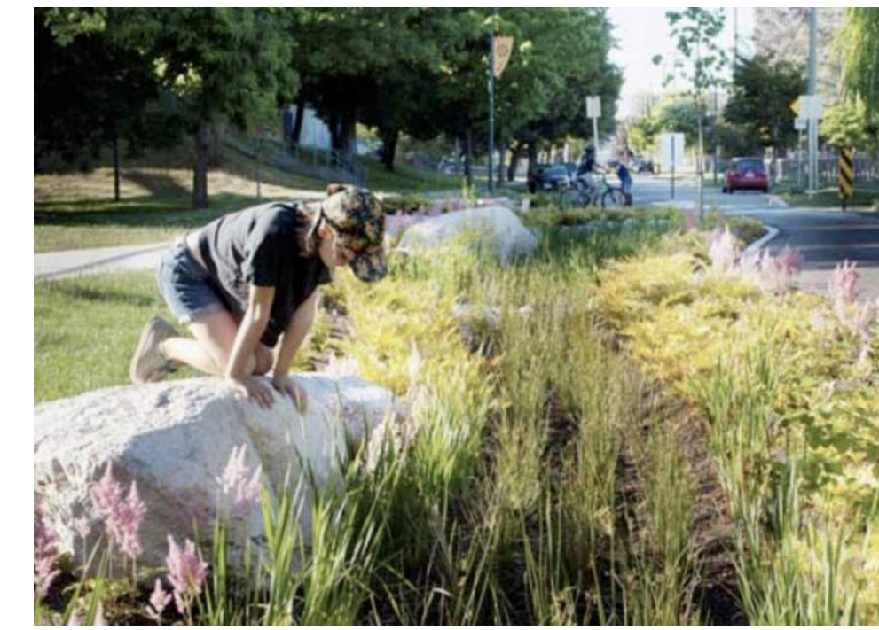
Rain Garden and Bioswale
