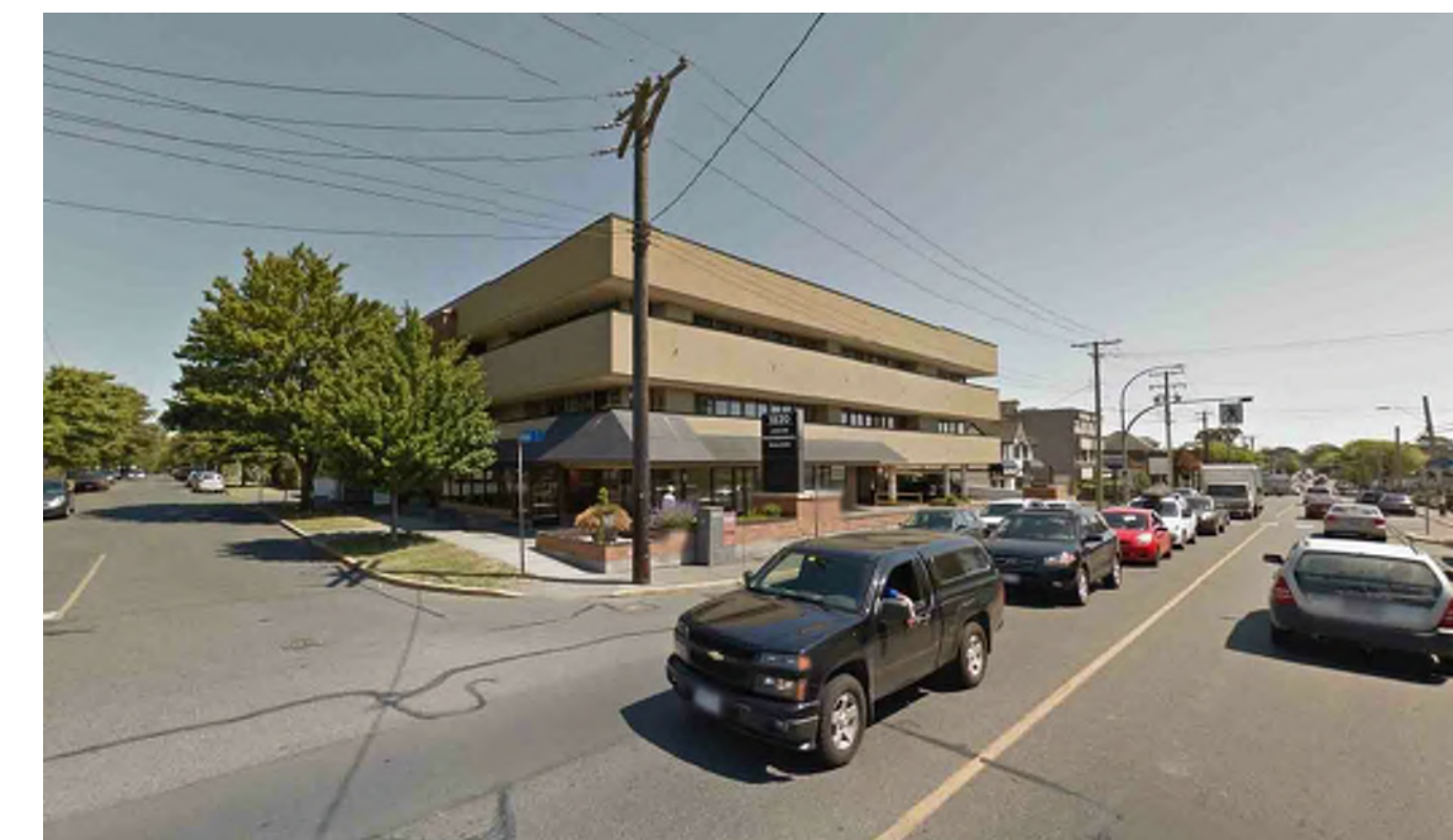
⑨ OPPOSITE STRUCTURE ON CORNER OAK BAY / BANK ST
