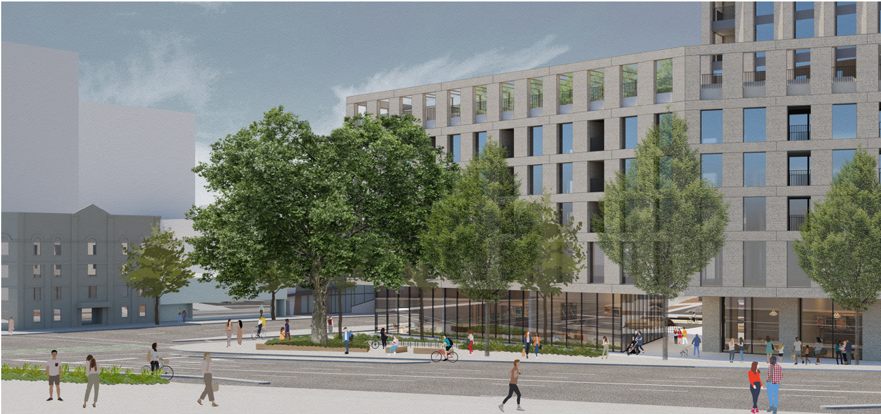
VIEW FROM BLANSHARD STREET LOOKING SOUTHWEST
