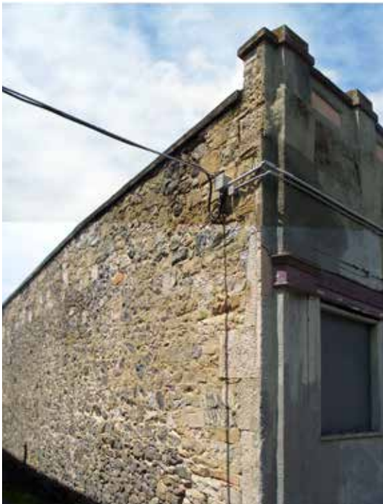
Current side and front elevations showing the stone construction with quioning on the corner.
