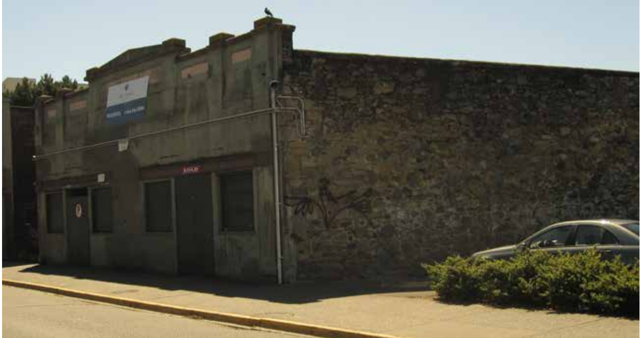
Current front elevation of Fraser Warehouse with later applied stucco.
