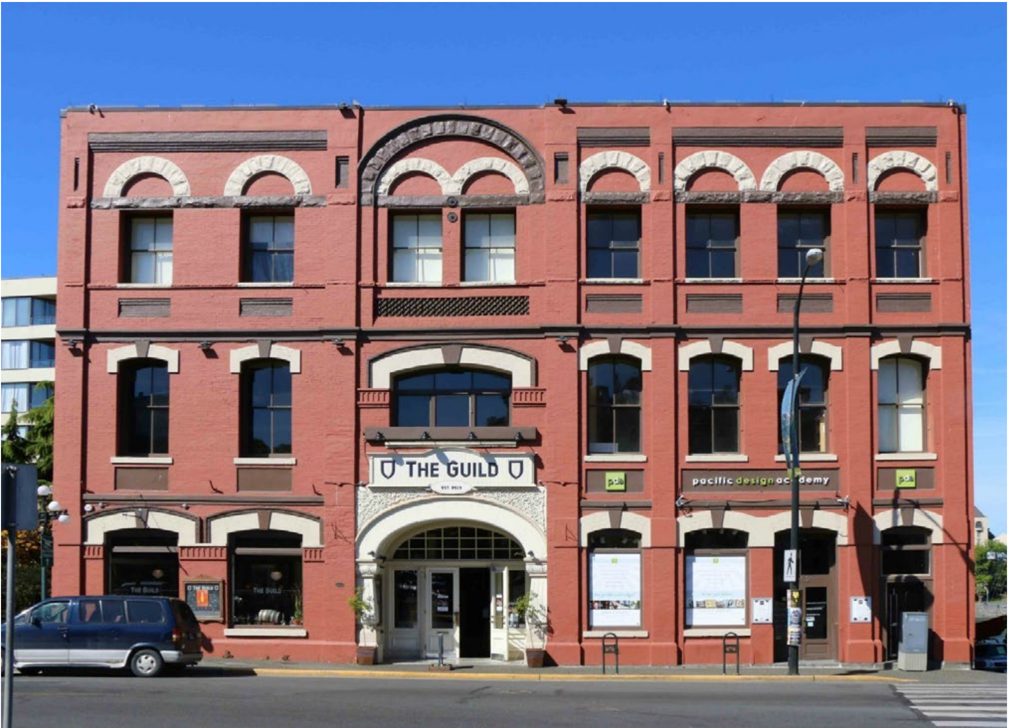
VIEW OF WHARF STREET FRONTAGE
