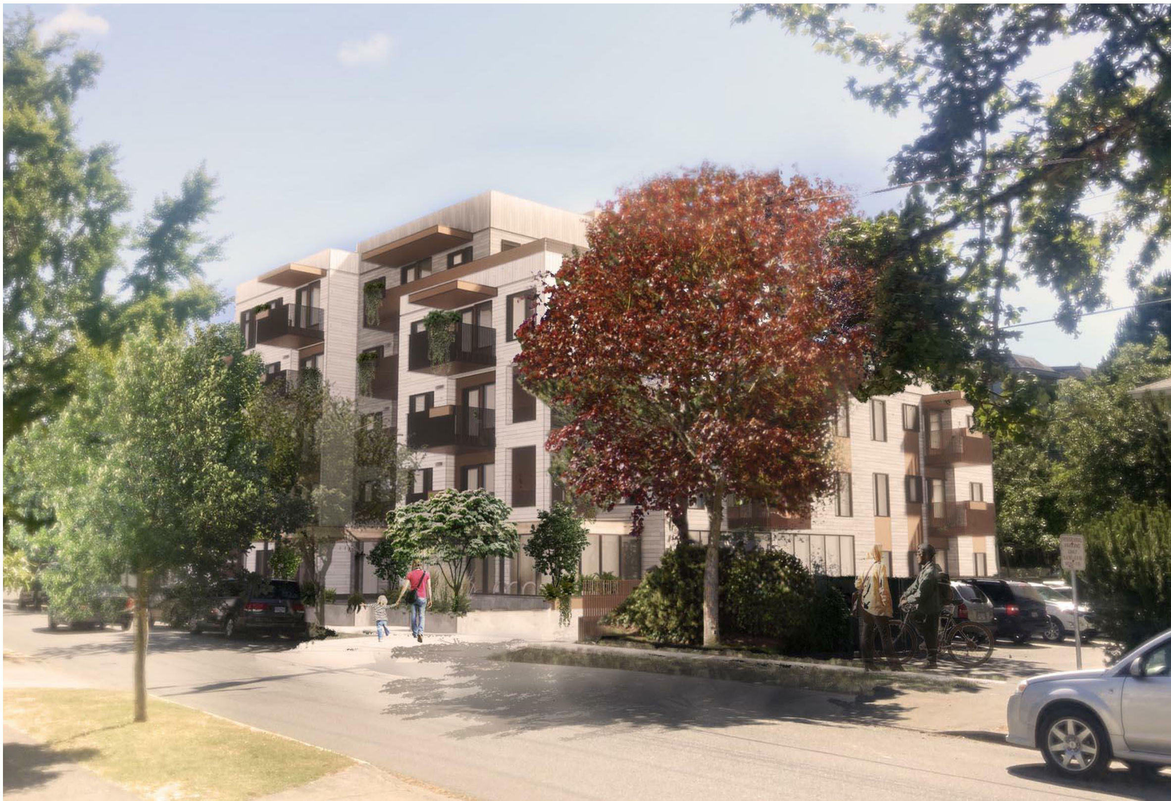
View from single-family yard across Camosun
