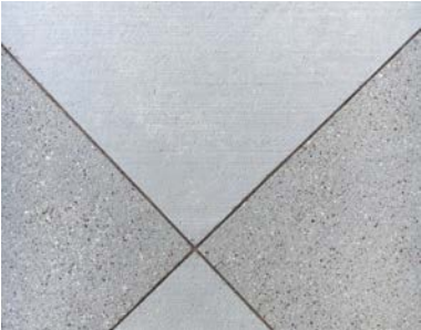
Cast-in-place Concrete (sawcut, non-slip)
