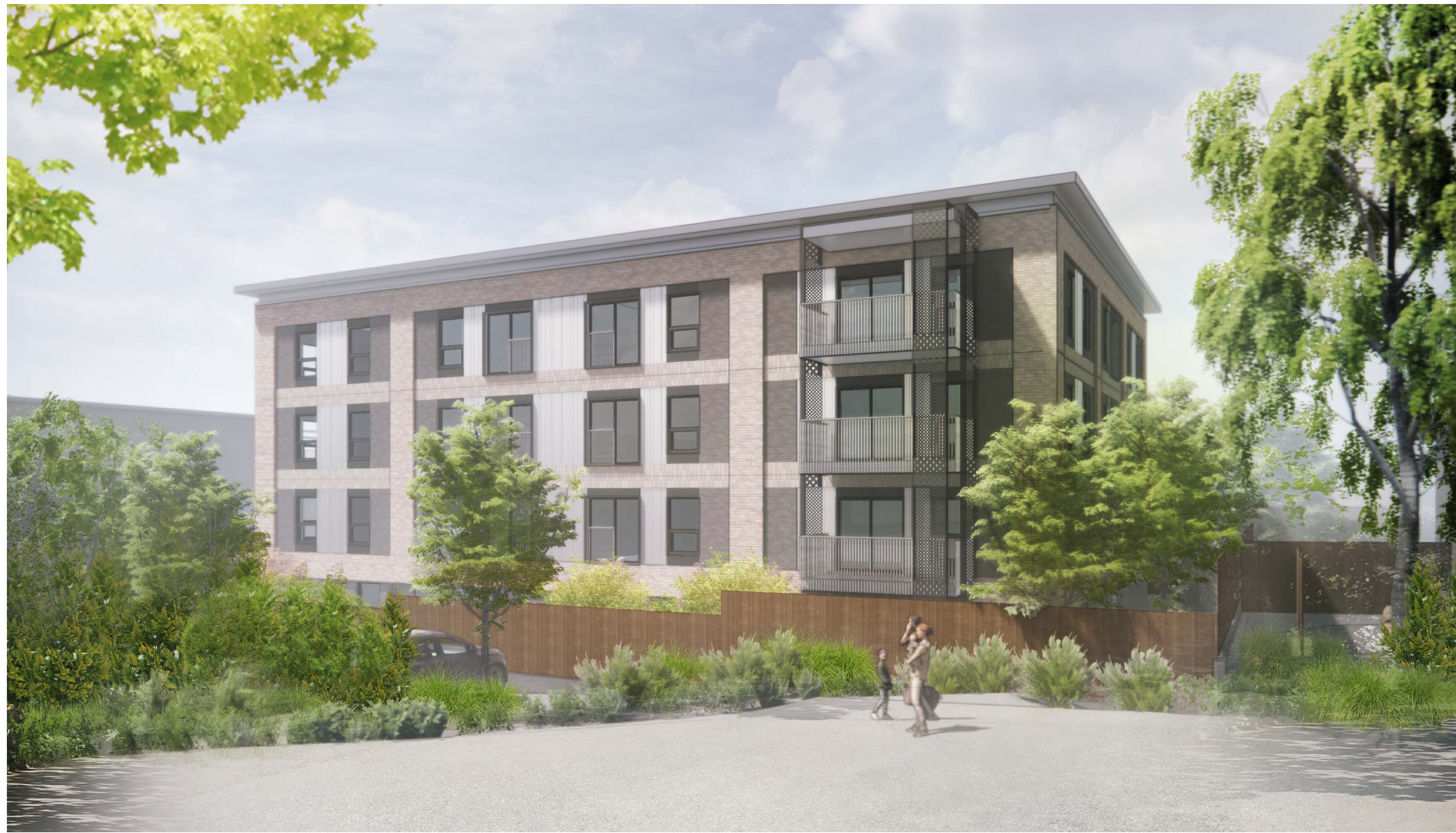
CLOSE UP VIEW FROM FREWING LANE
