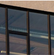
Windows Fibreglass frames and clear Low-E glass Colour: Black
