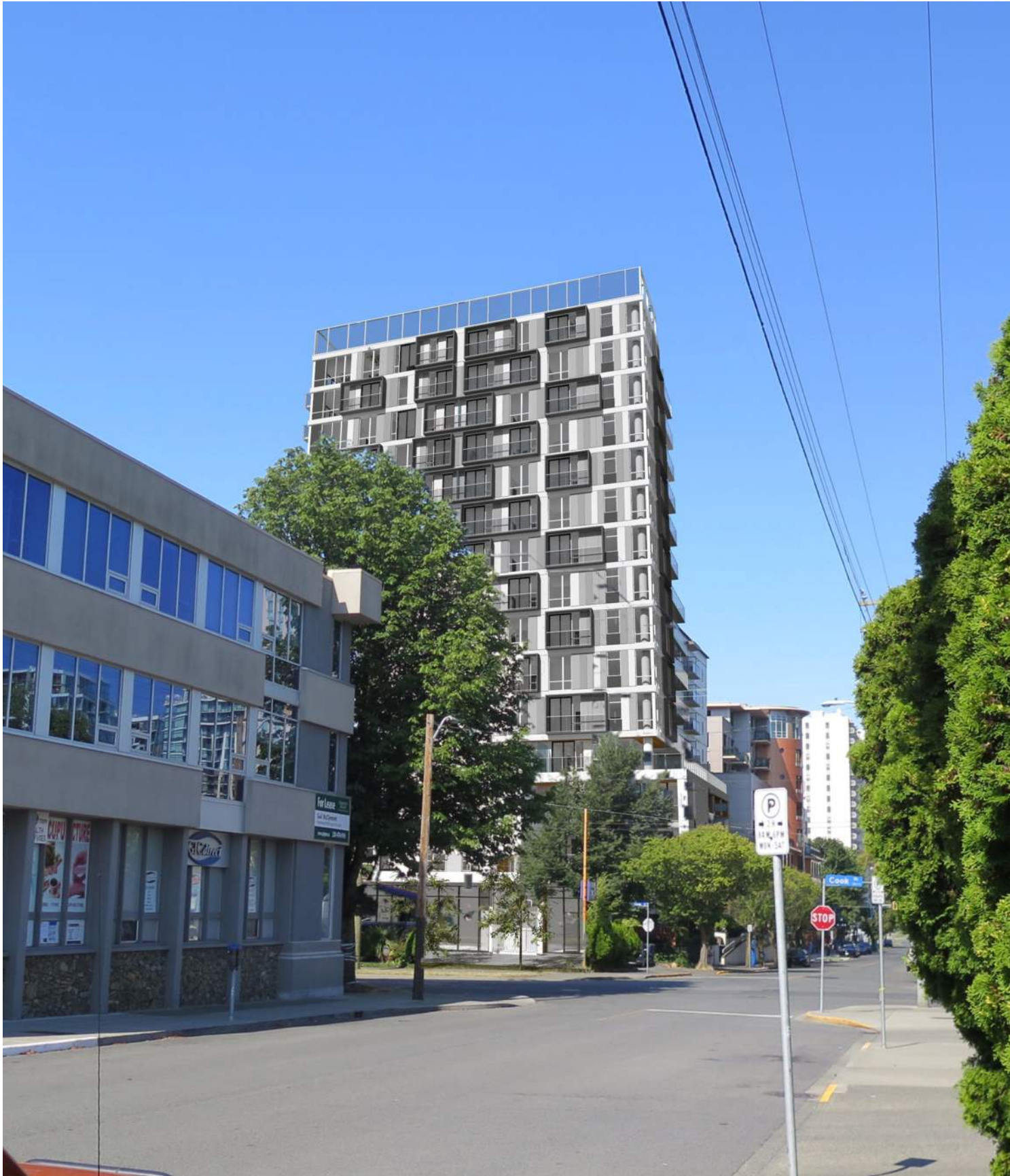
D View Street Looking West
