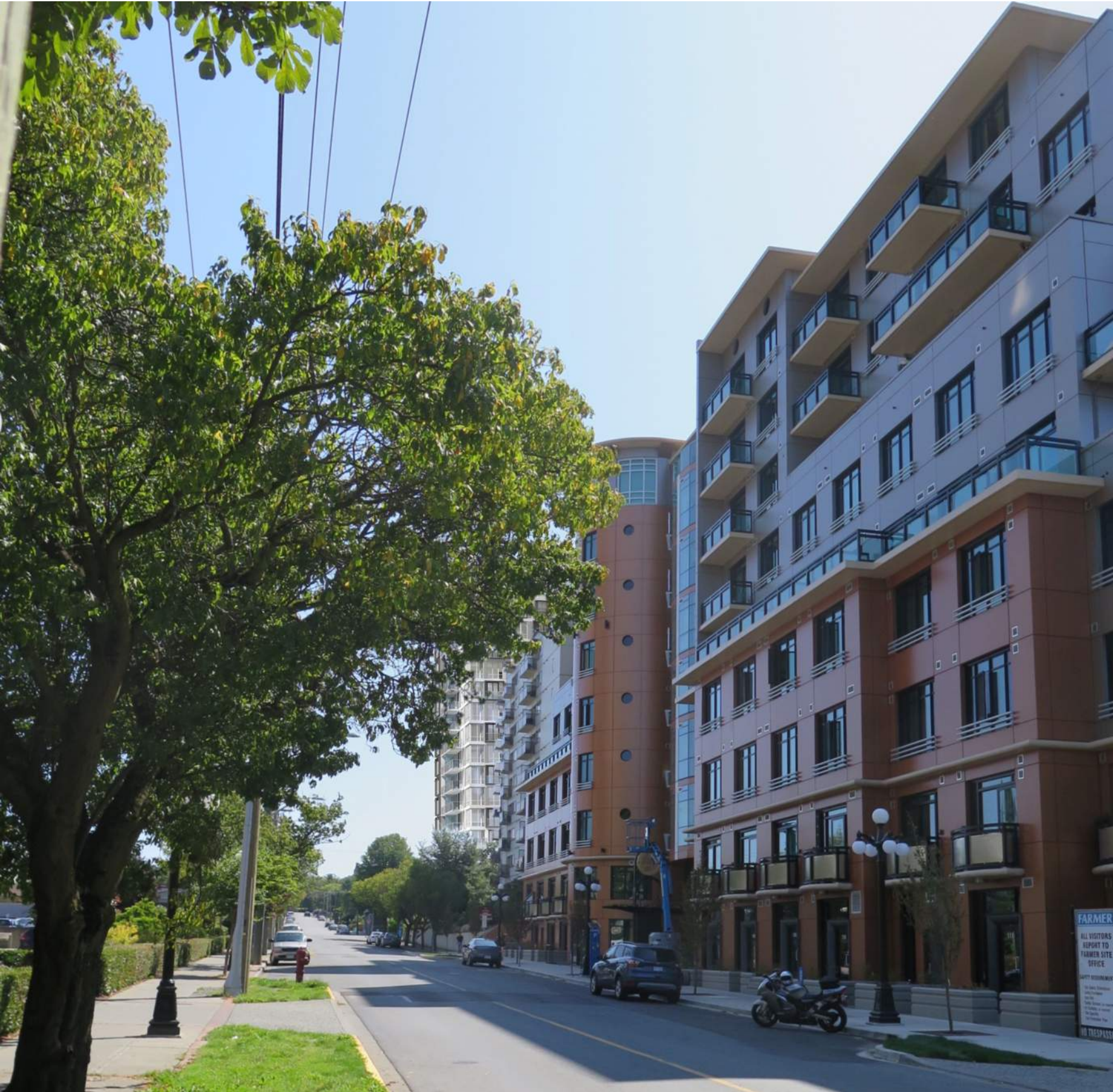
B View Street Looking East
