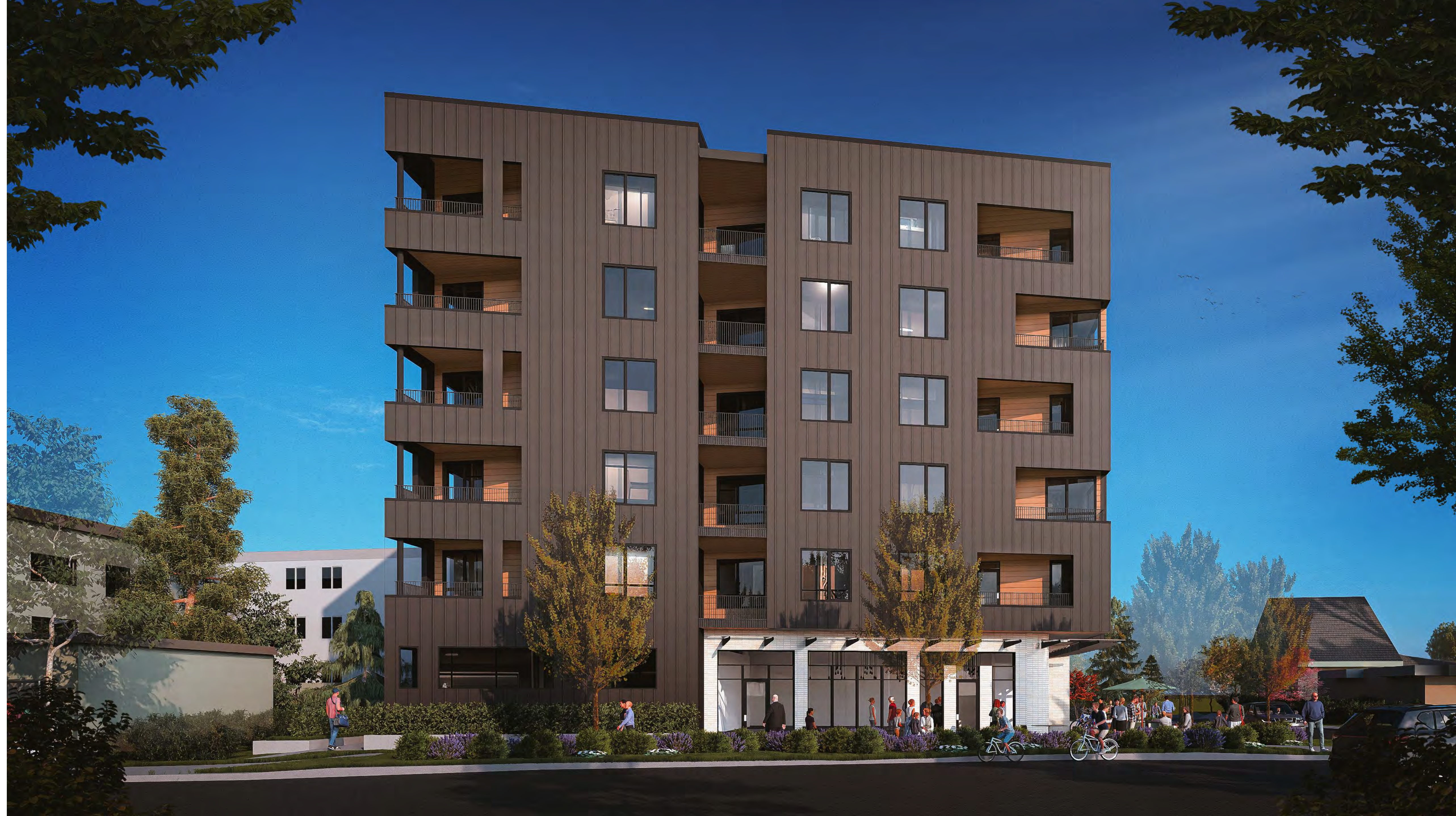
North Elevation - Fort St
