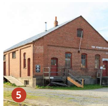
Stores building, view from east (Focus Equities)
