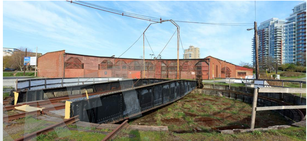
Roundhouse, Back Shop, and Turntable at Bayview Place Site, 2020 (Focus Equities)
