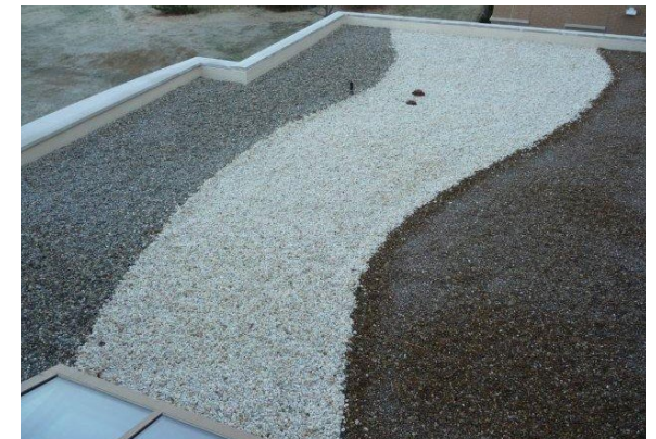
Roof treatment using light and reflective colours to minimize urban heat island effect
