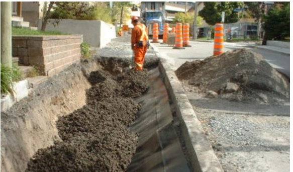
Structural soil installation
