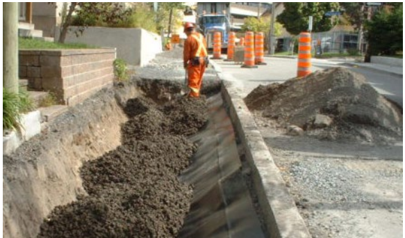
Structural soil installation
