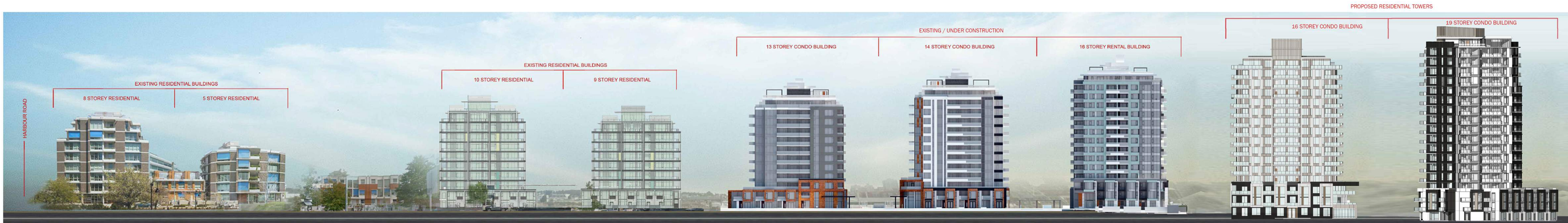
WEST SIDE STREETSCAPE (TYEE ROAD)
