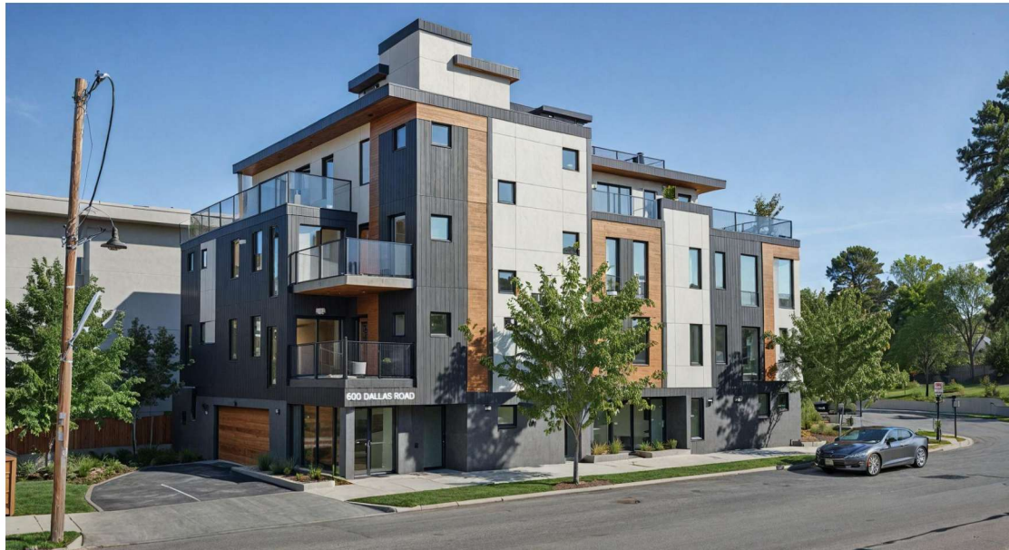
VIEW OF PROJECT FROM GOVERNMENT STREET
