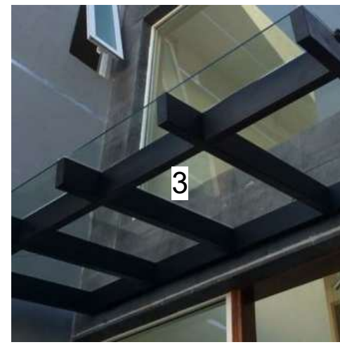
Glass/Metal Entrance Canopy
