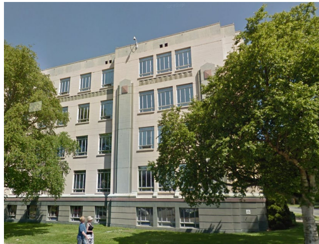
Figure 19: Douglas Building Southwest Front Elevation
