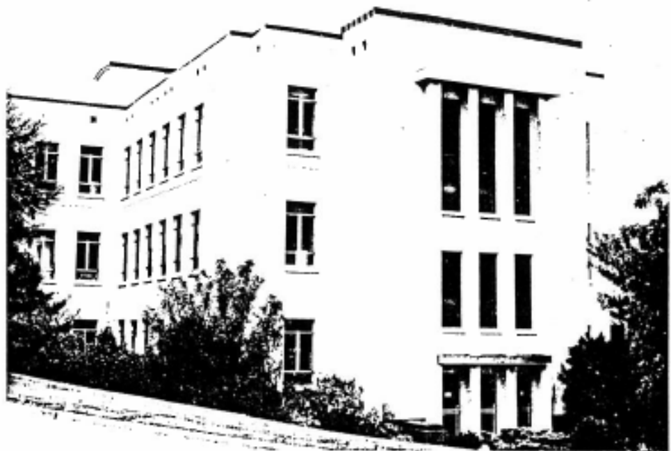
B.C. POWER COMMISSION BUILDING 780 BLANSHARD STREET H. Whittaker, Chief Architect, Provincial Department of Public Works, 1939-1940
