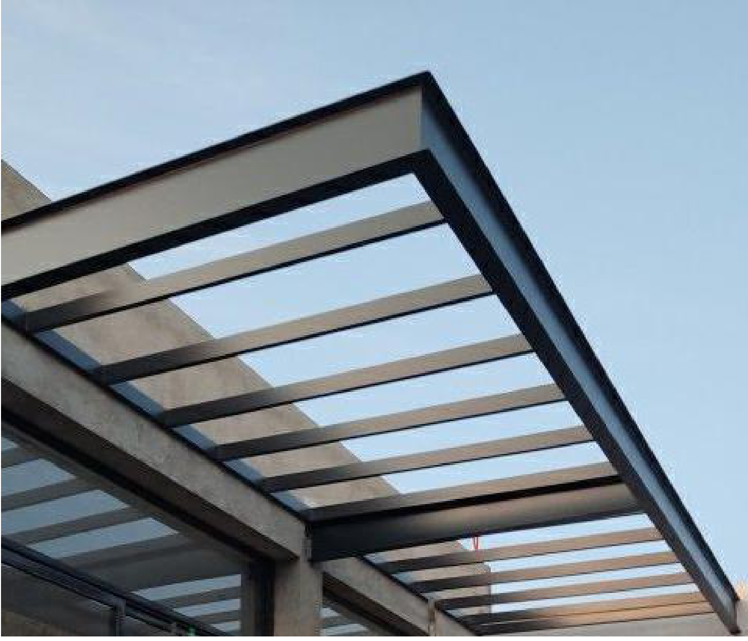
BLACK PAINTED STEEL CANOPY W/ LAMINATED GLAZING
