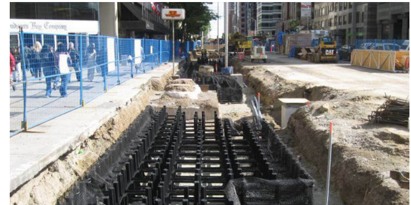
Soil cell installation
