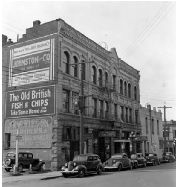
Duck's Building, 1318-1322 Broad Street, 1947. [Daily Colonist. City of Victoria Archives M08633]
