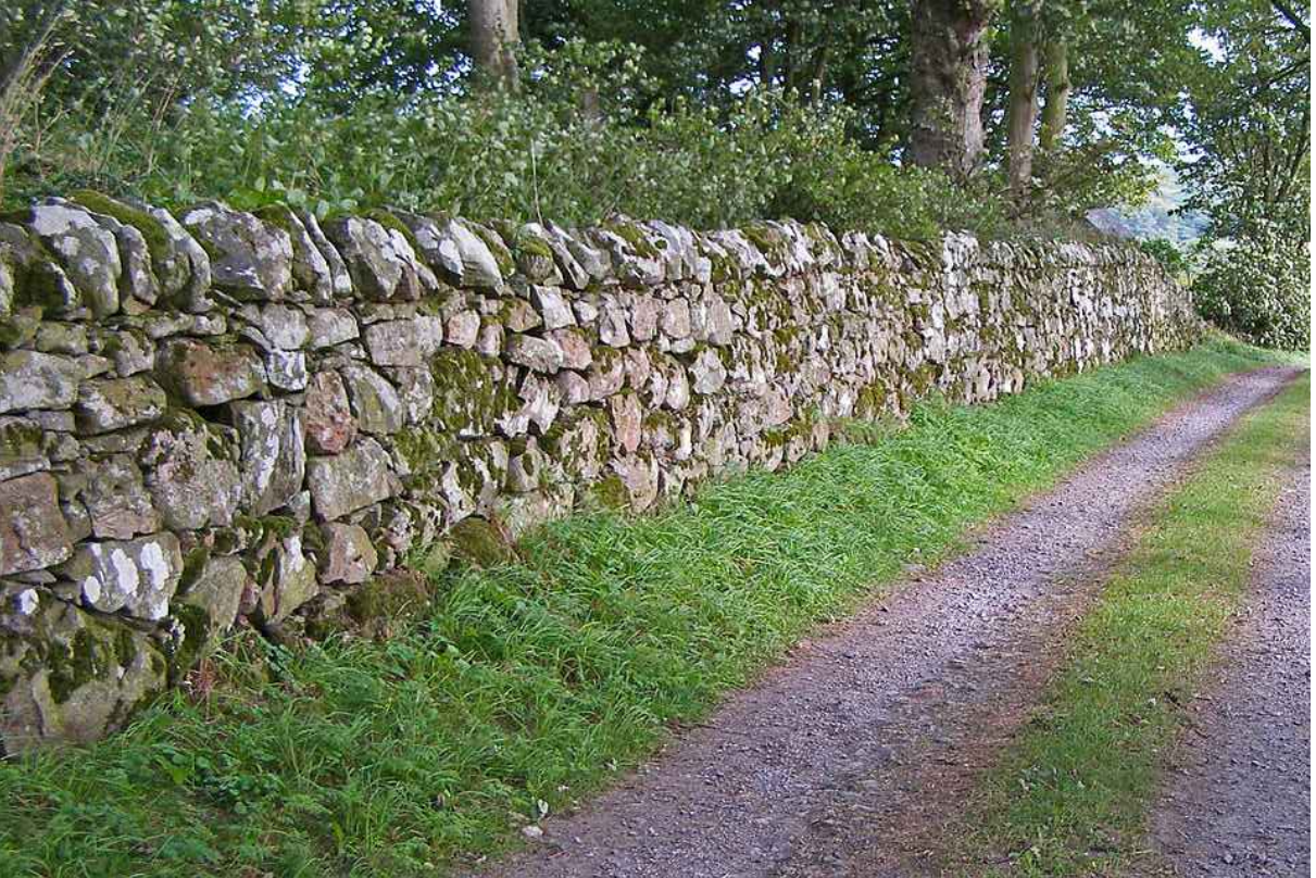
GRANITE STONE WALL PRESERVATION
