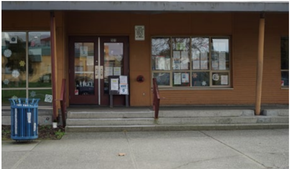
Quadra Village Community Centre
