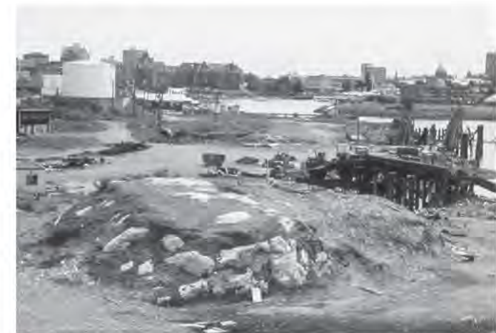
Site looking east, 1983
