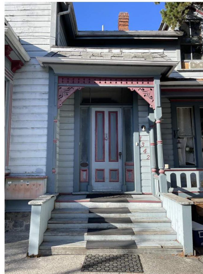
EXISTING FRONT ENTRY
