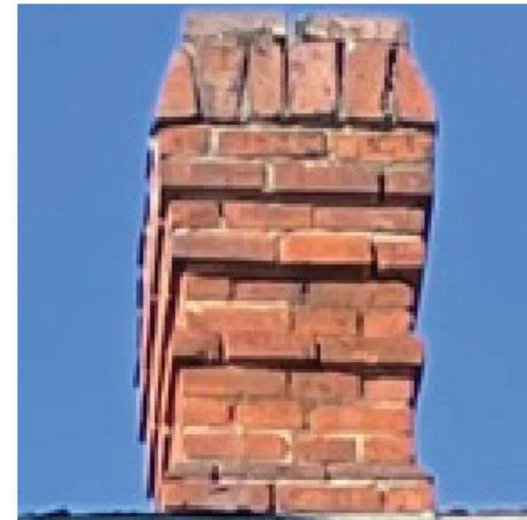
B1 EXISTING BRICK
