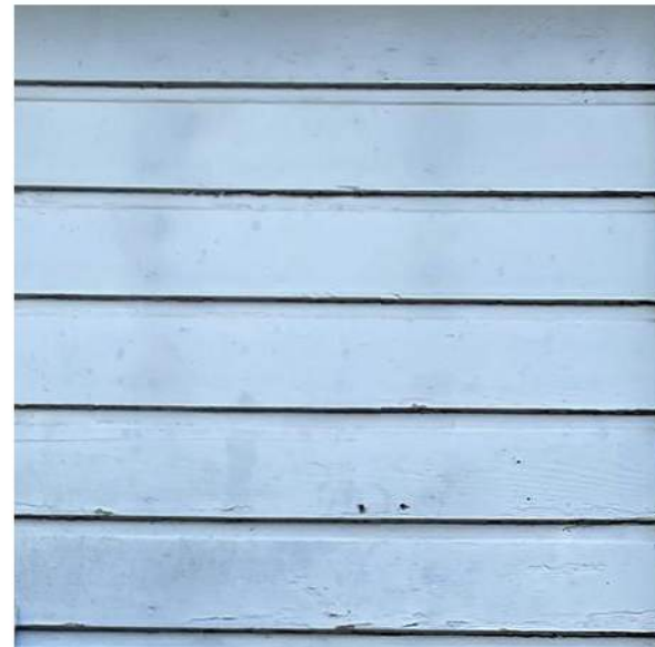
S1 EXISTING CHANNEL RUSTIC SIDING
