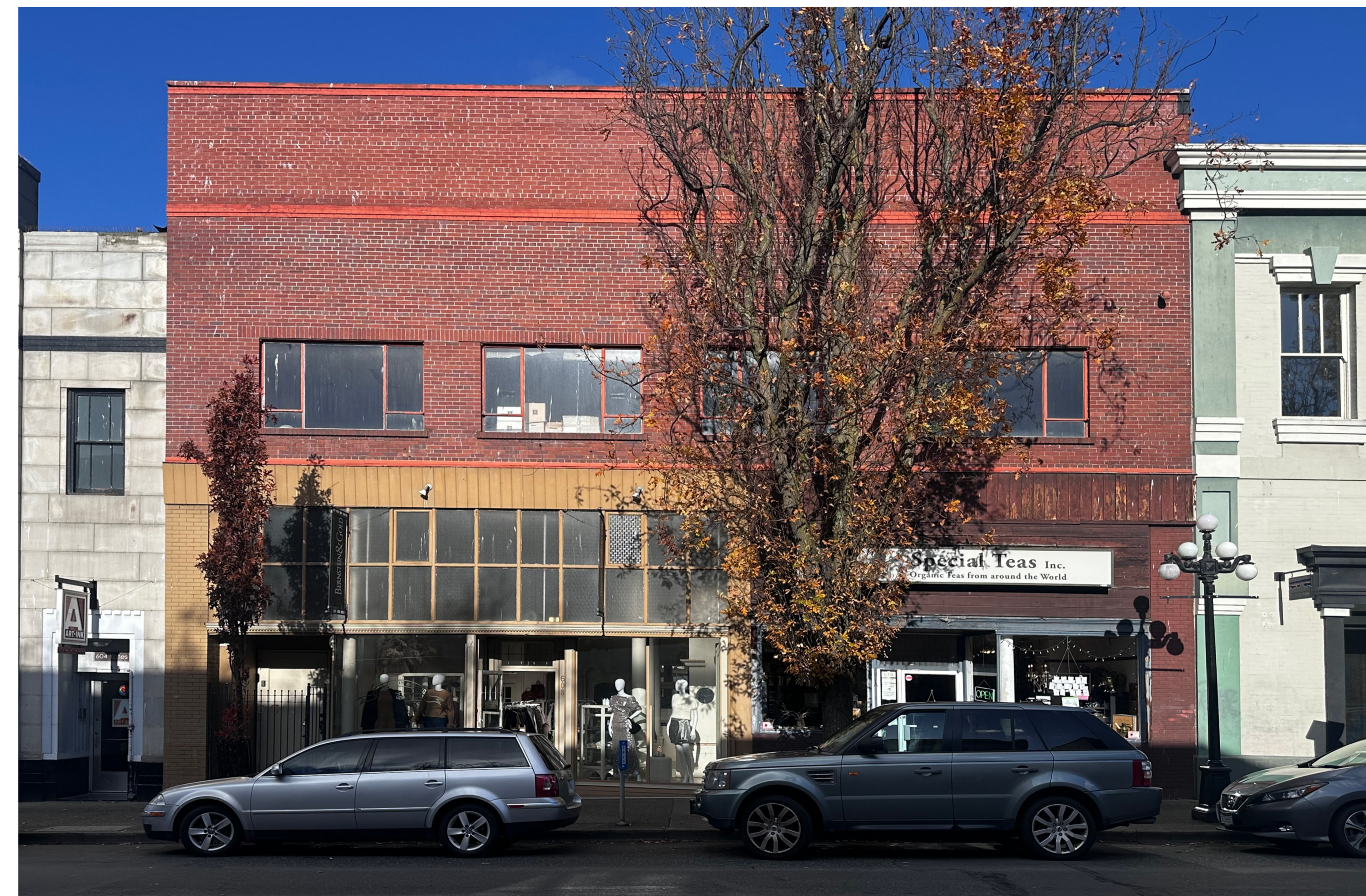
1 Photograph Of Existing Elevation 5K-04 Scale: 1/4" = 1'-0"
