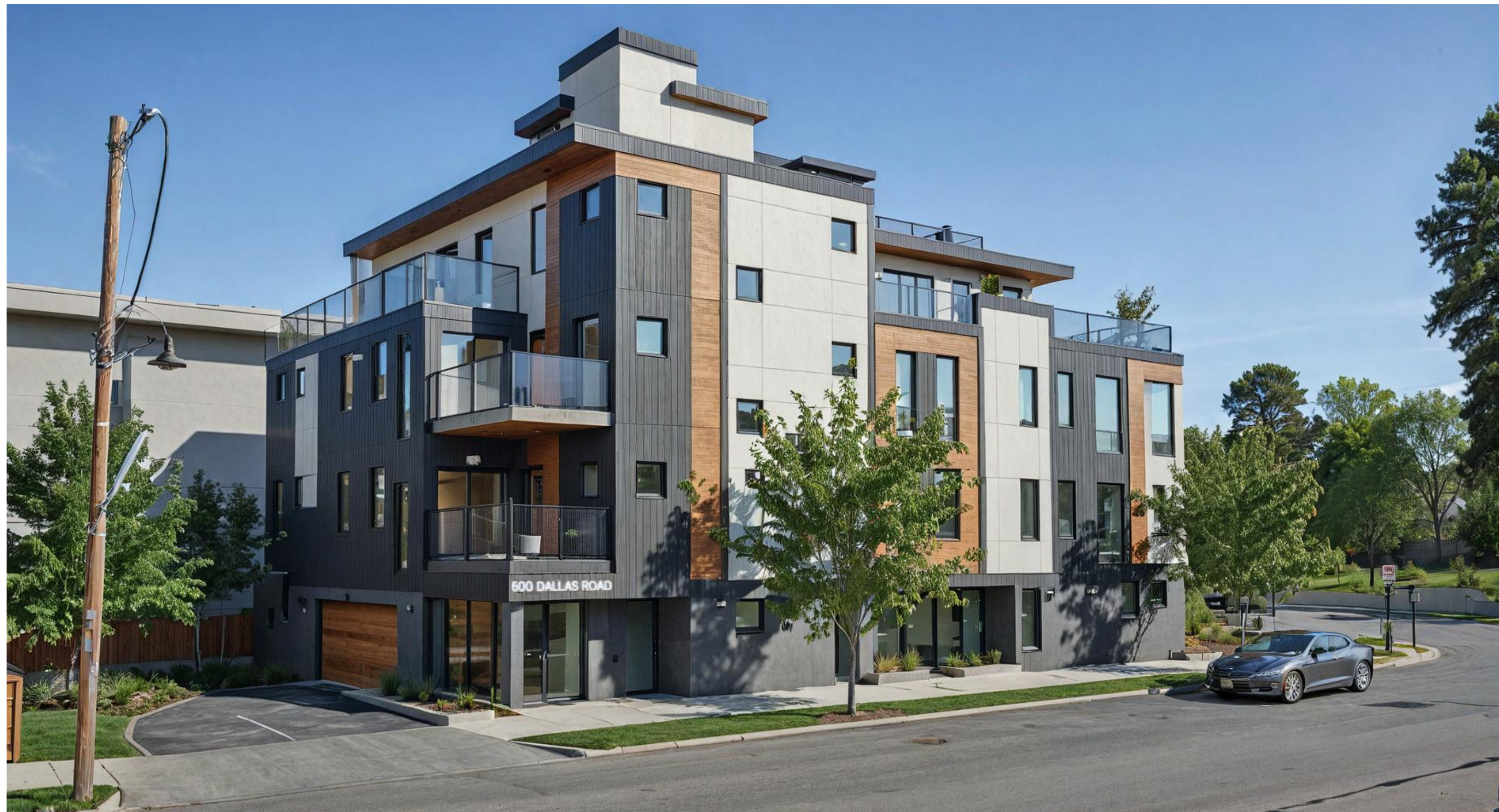
VIEW OF PROJECT FROM GOVERNMENT STREET
