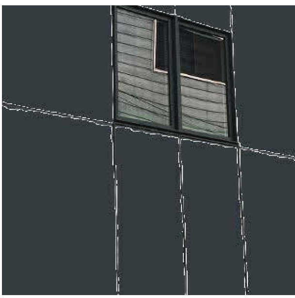
(3) ALUMINUM SANDWICH PANELS COLOUR: ANTHRACITE
