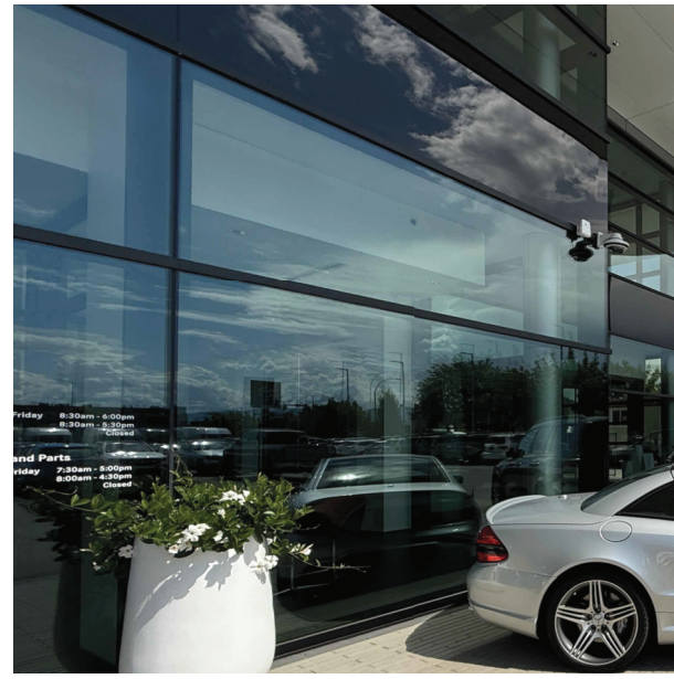
(1) ALUMINUM STOREFRONT WINDOW/DOOR COLOUR: CHARCOAL
