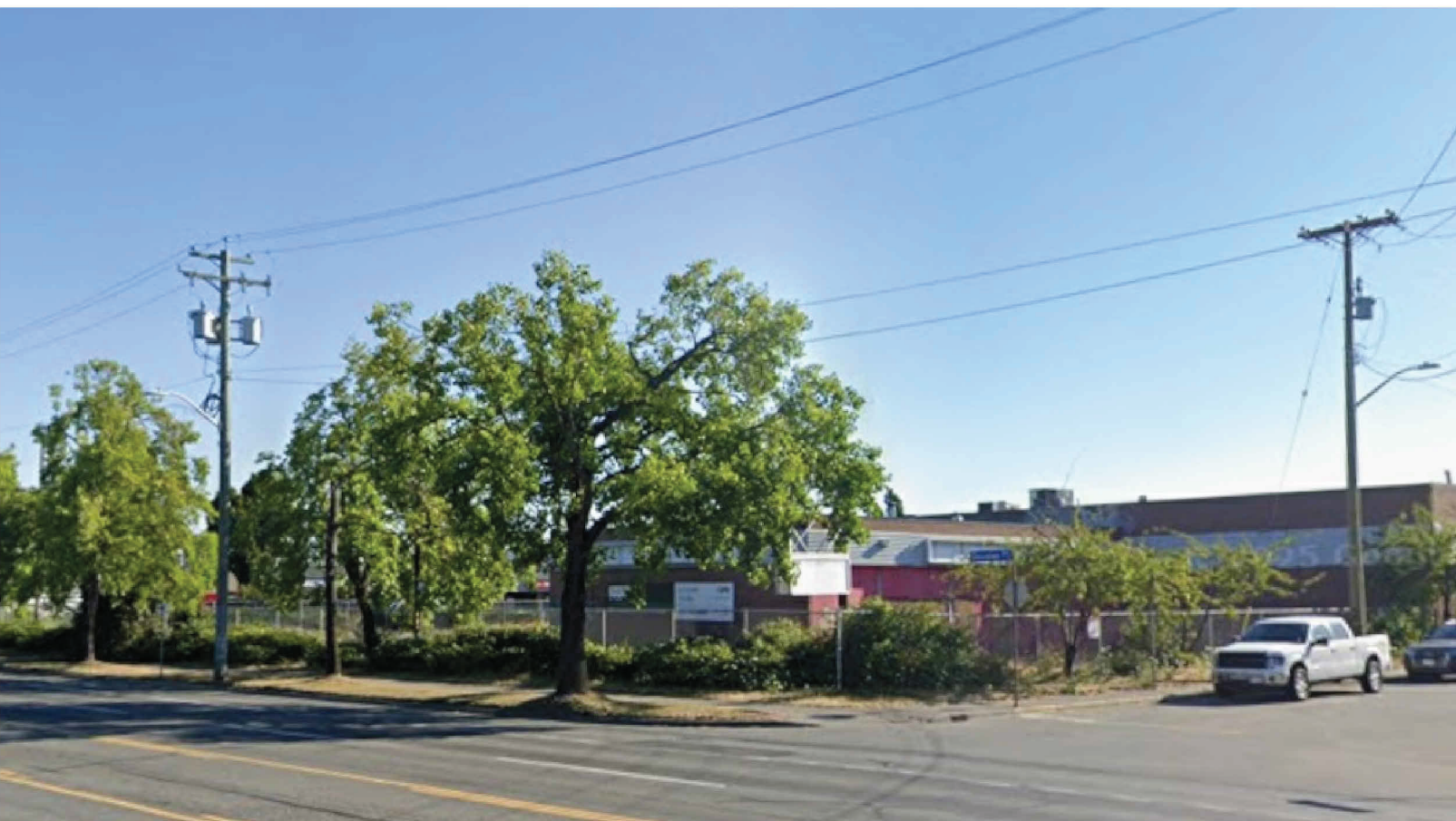
EXISTING STREET VIEW
