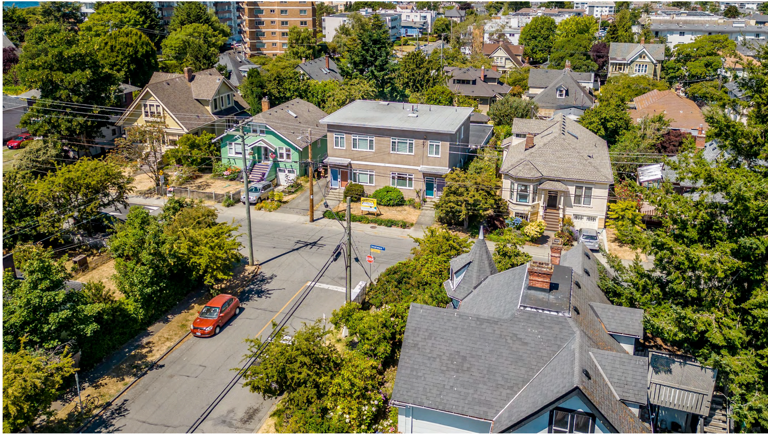
1 Existing Building, 50 Government
