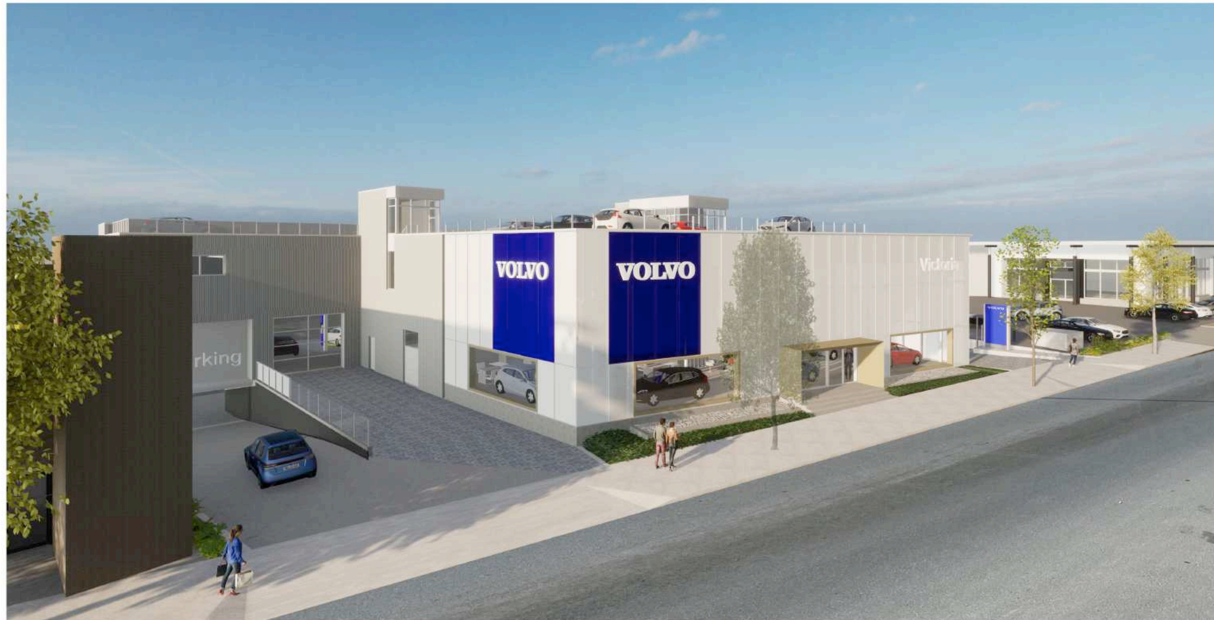
1 Aerial Street View Looking North West
