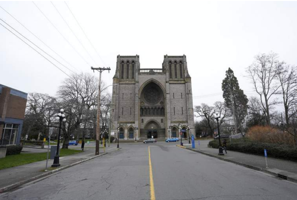
1. Courtney Street, looking east
