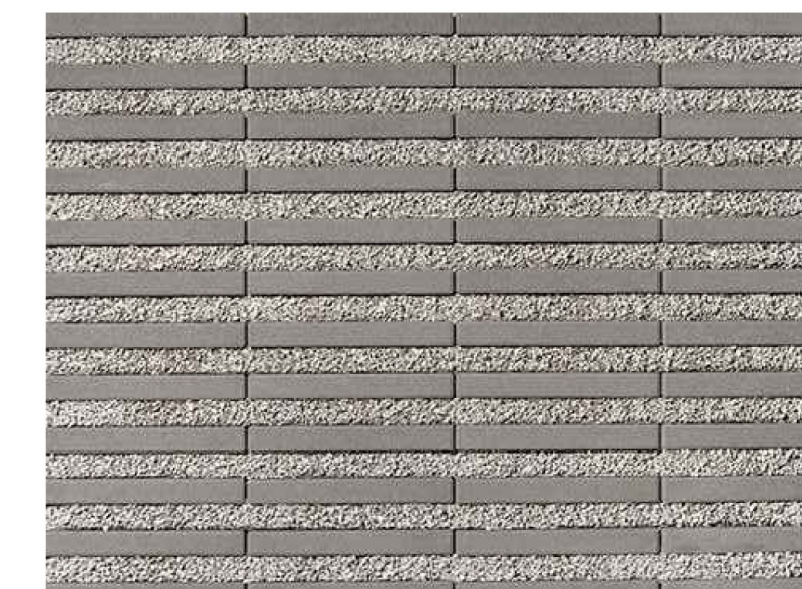
PERMEABLE PAVER DRIVEWAY
