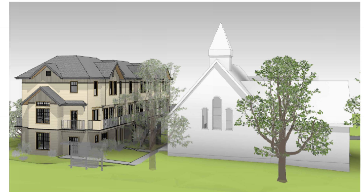
5 VIEW FROM COOK STREET
