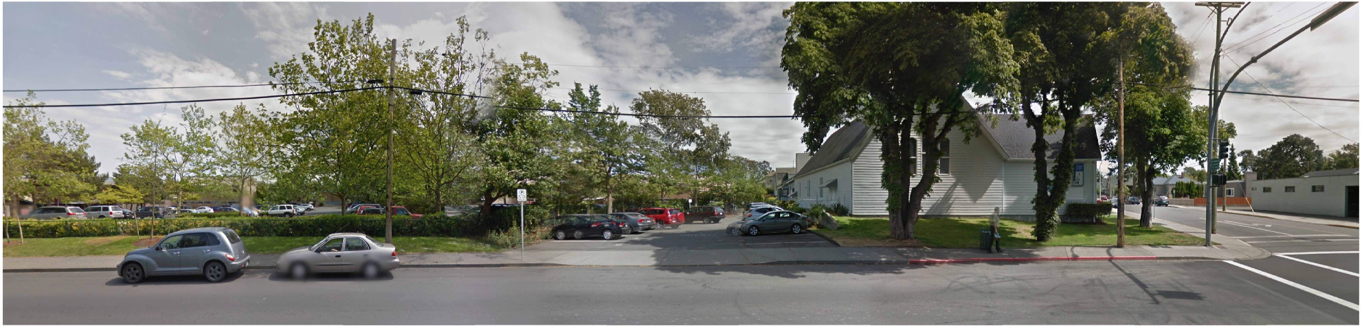
COOK STREET VIEW - EXISTING
