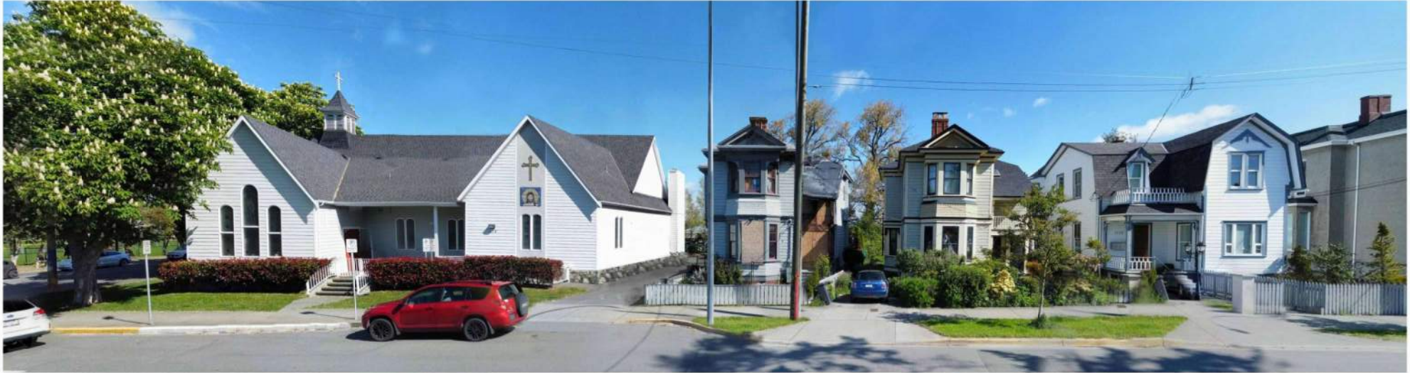
CALEDONIA STREET VIEW - EXISTING
