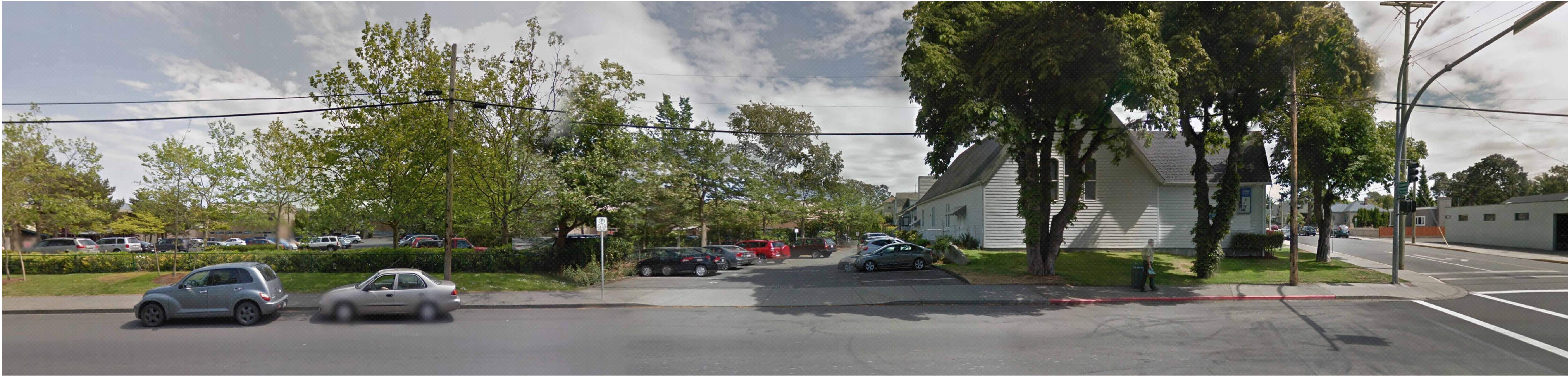
COOK STREET VIEW - EXISTING
